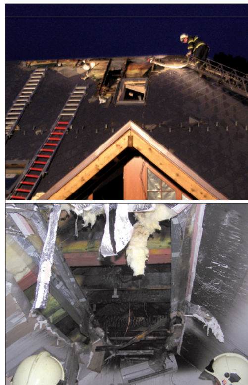
Fig. 2 Burning-in of the hotel's attic
